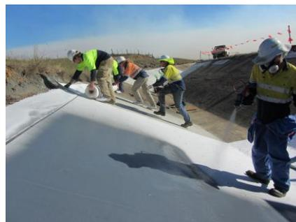
Figure 2. Open Concrete Water Supply Channel DURING remediation with Geofabric and Tufflon polyurea
