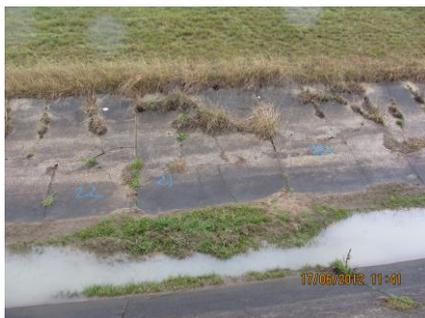
Figure 1. Open Concrete Water Supply Channel BEFORE remediation with Geofabric and Tufflon polyurea
