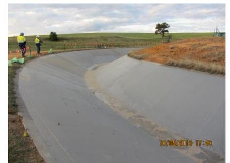
Figure 3. Open Concrete Water Supply Channel AFTER Remediation with Geofabric and Tufflon polyurea
